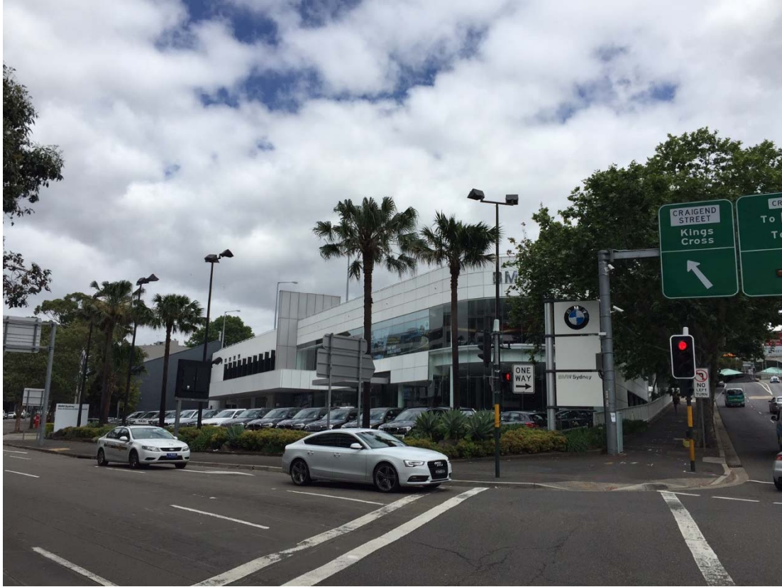
Figure 3: McLachlan Street frontage, viewed from the north-east
