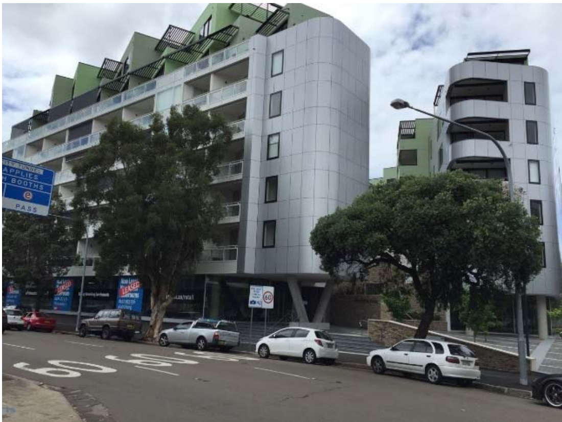
Figure 10: Northern portion of Advanx development, to the east of the site on the opposite side of McLachlan Avenue
