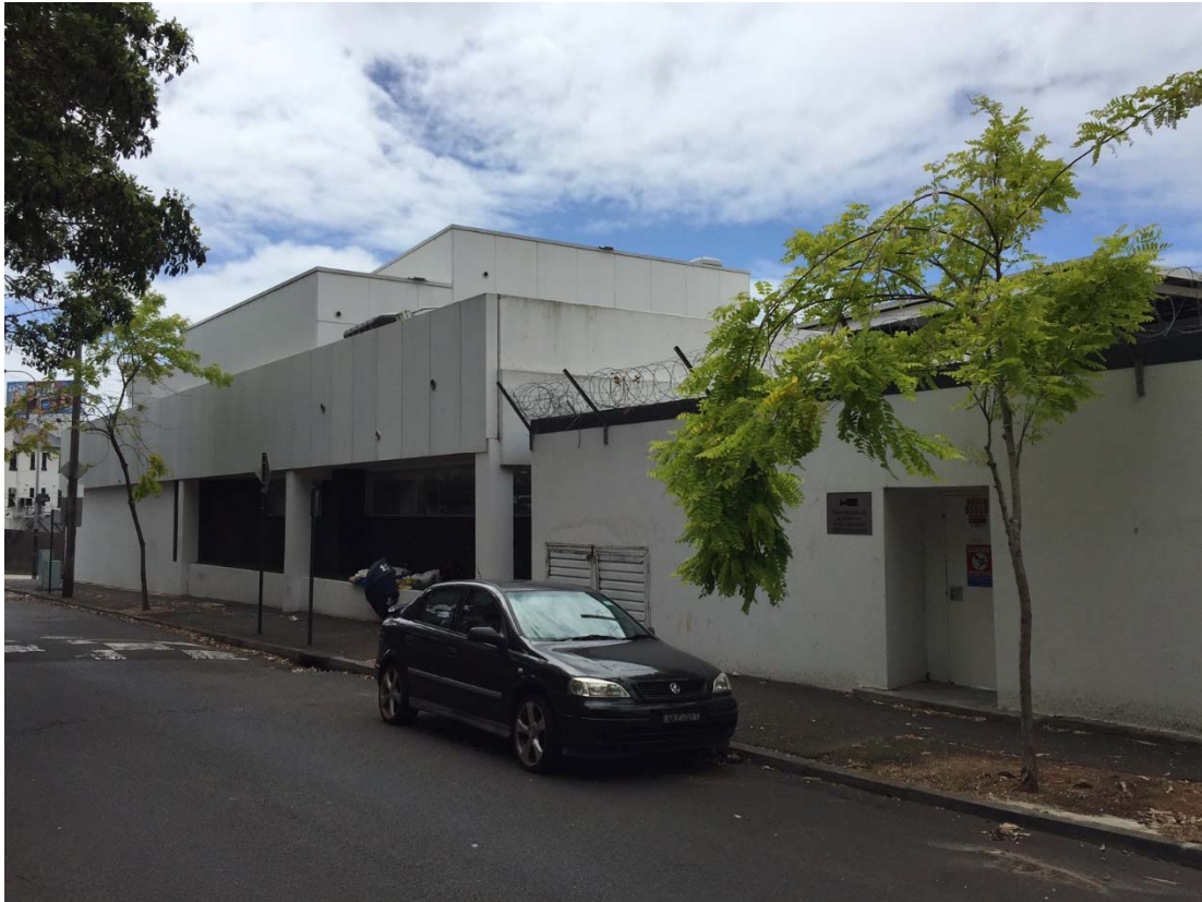
Figure 5: Barcom Street frontage close to the intersection with Craigend Street
